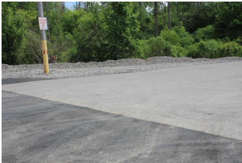
This berm next to the driveway and Donner Creek is 10" to 24" high
