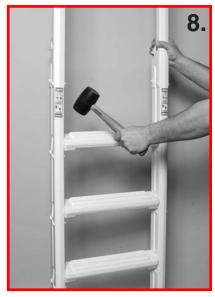
Tap the treads downward so that they seat fully into the bottom of the keyhole slots.
