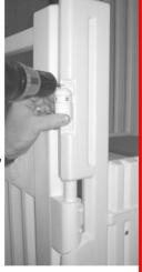
ADJUST THE TENSION ON CLOSER (See details provided on closer Package) SO THE GATE WILL SELF CLOSE AND LATCH EVERY TIME. CLOSE THE GATE SEVERAL TIMES AND MAKE ADJUSTMENTS IF NECESSARY.
