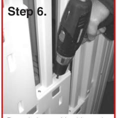
Fasten the bottom of the pickets to the step unit at the pre-marked locations using twelve (12) #10 x 1-1/4" screws.
