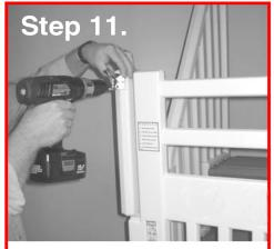
Install the latch to the upper mounting block of the latch mounting post using four (4) #10 x 1-1/4" self tapping screws.
