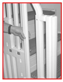
Align one of the triple pickets into the notches of the handrail at the top of the unit. Fasten the pickets in place, at the top of the pickets, using the  $\#10 \times 3/4$ " screws. Continue placing and fastening the double pickets and then the single picket. Repeat for the opposite handrail. Cover the ends of the screws with the protective caps.
