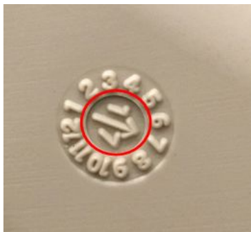
Photo 4: The two numbers in the middle next to the arrow represent the year of the manufacturing/date code. (Years 2013-2018 are recalled.)
